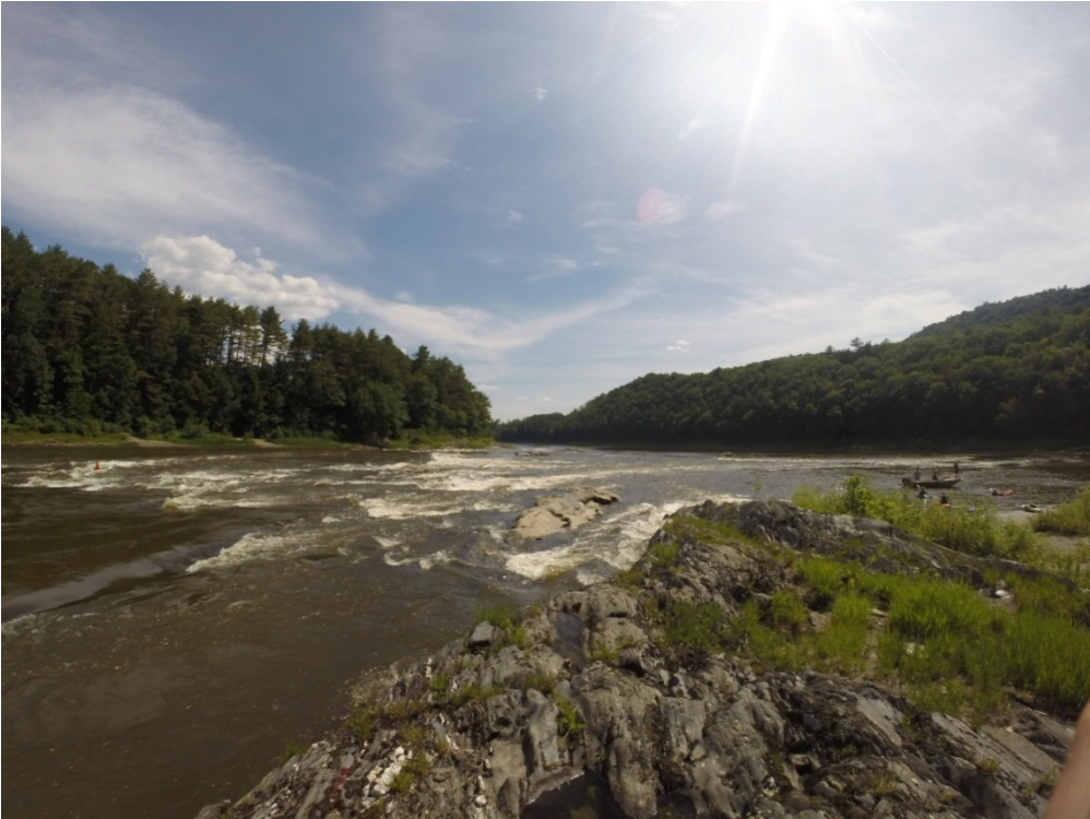
6,750 cfs – Right center slot washed over
