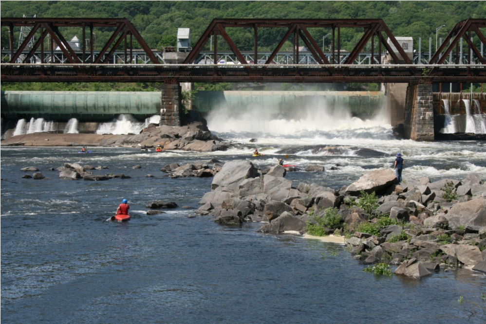
3,300 cfs – Dome rock feature near spillway
